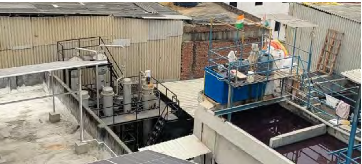
Overview of MEE and ETP area
